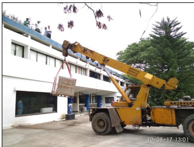
Panel unloading at NCL rooftop
