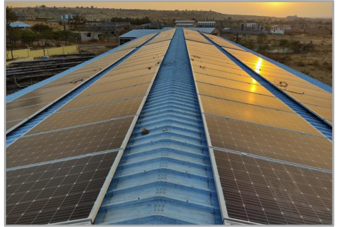
On workshop roof
