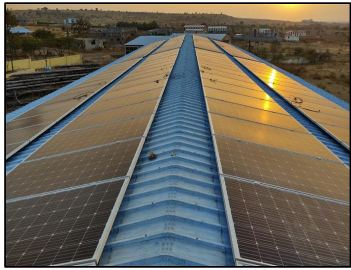
On workshop Roof
