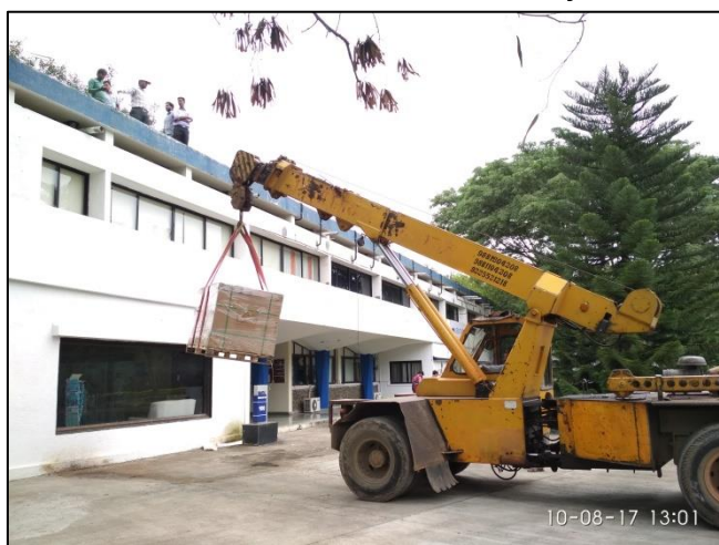
Panel unloading at NCL rooftop
